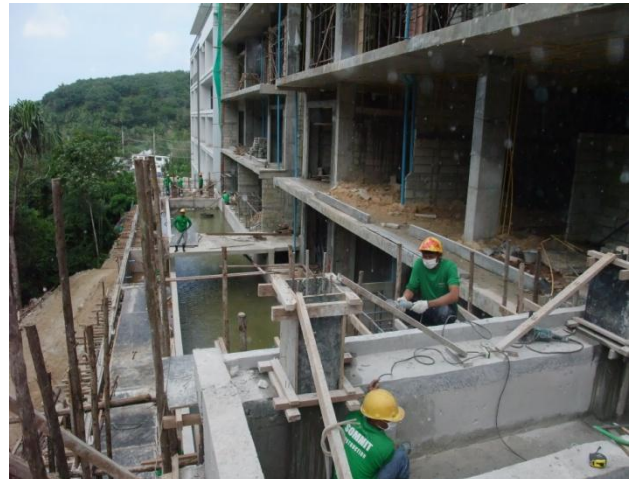
All swimming pool foundations of C Phase structure completed
