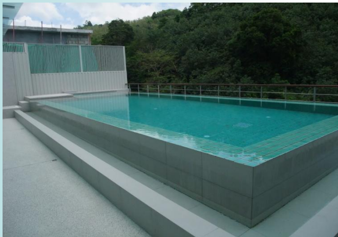
Penthouse C1 pool and Jacuzzi – unit completed
