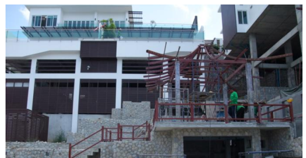
Rock pool, gazebo and fountain outside gym near completion
