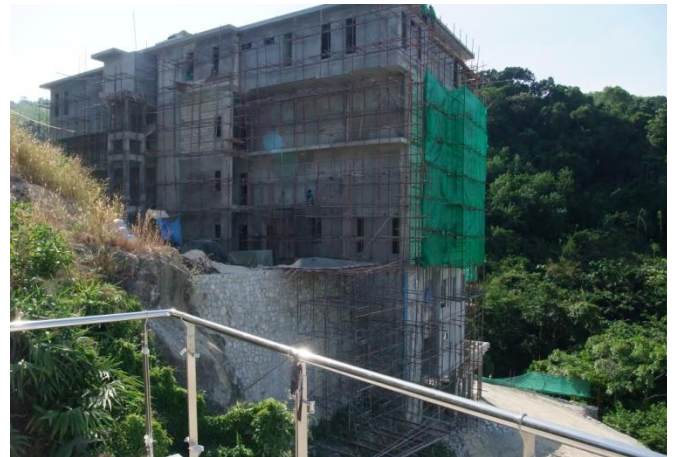
Building C1 – completing external rendering
