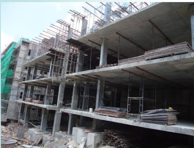
C Phase – Building C2 preparing for 4 th floor level
